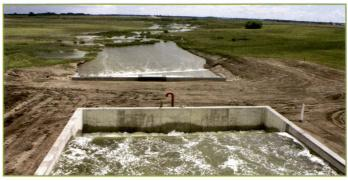
Water Commission, and is designed to prevent a potentially catastrophic overflow if the lake rises to the natural overflow elevation. Discharge through the structure is controlled by stop logs which are kept approximately one foot below the lake elevation.
