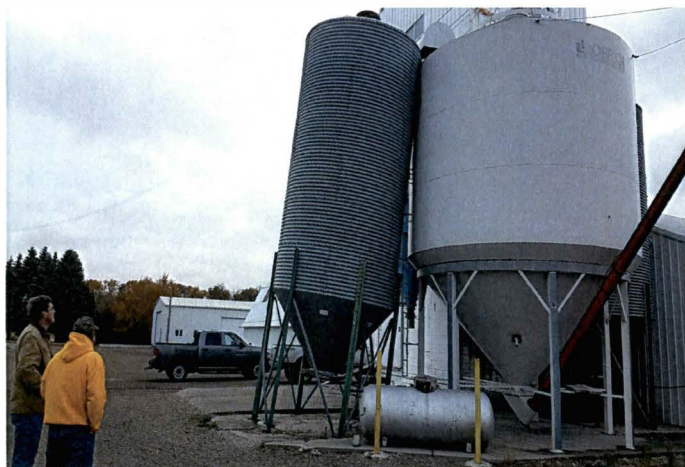
Old Holding Bin—Result of Failed Concrete
