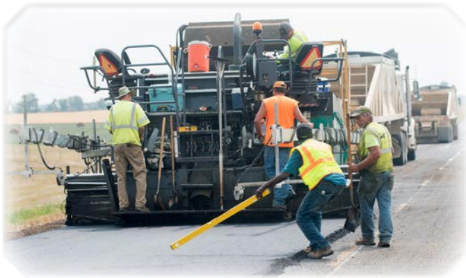
Resurfacing a highway in Dickinson District.
