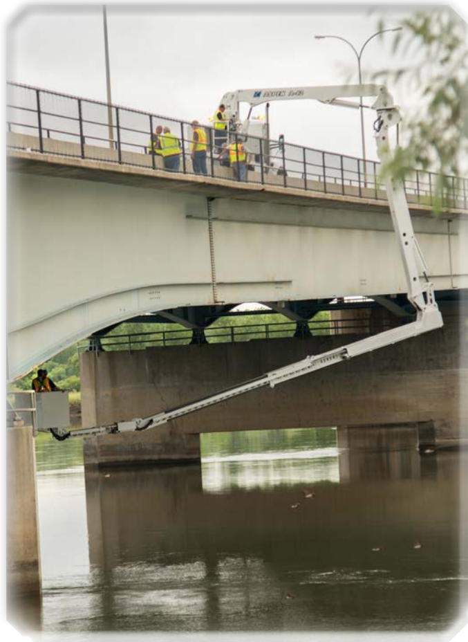
Bridge Inspection equipment on Expressway Bridge in Bismarck.
