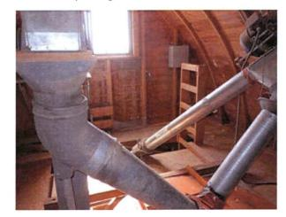
5<sup>th</sup> Floor-Main leg-Top of distributor-Accessible only by ladder-Note duct tape on legs
